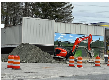
Flat Roof (inconsistent)
