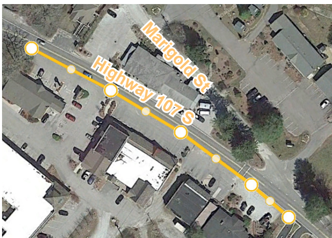
Lack of definition between driveways and roadway along this 477 foot long stretch of Hwy 107 S makes for an uncomfortable pedestrian environment.
