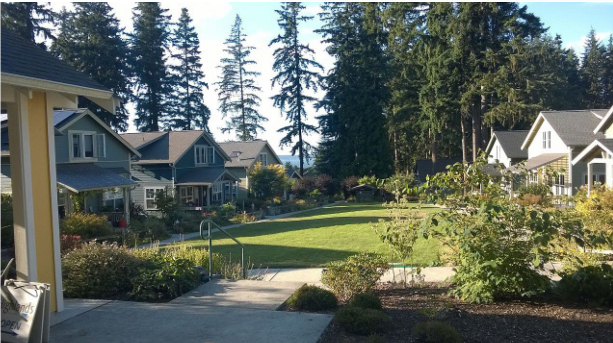
A pocket neighborhood in Langley, Washington includes cottage homes oriented around a shared green. This type of development could fit well into the existing character of Cashiers and also appeal to a broader demographic looking for low-maintenance seasonal homes or less expensive "missing middle" housing. (Image Source: Wikimedia Commons)
