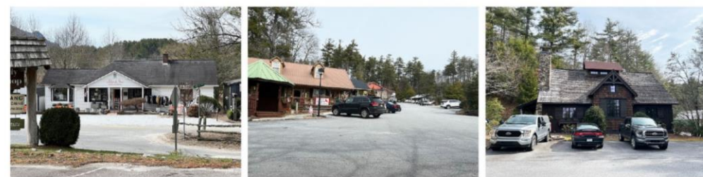
Common non-residential roofing materials in Cashiers
