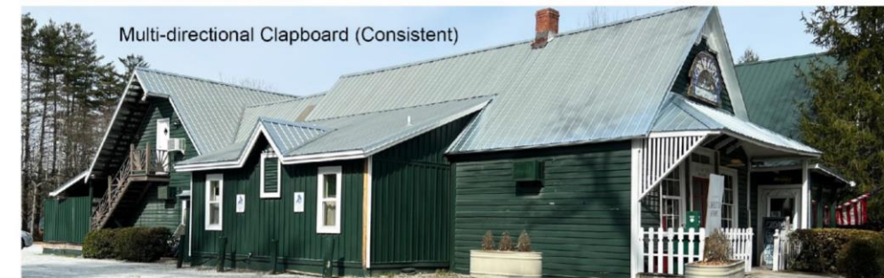
Common siding materials in Cashiers
