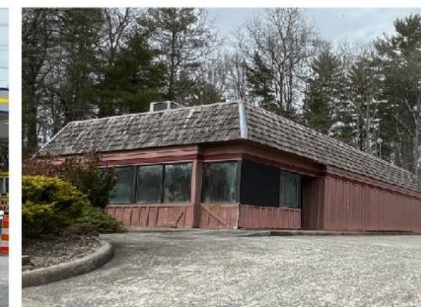
Mansard Roof (inconsistent)
