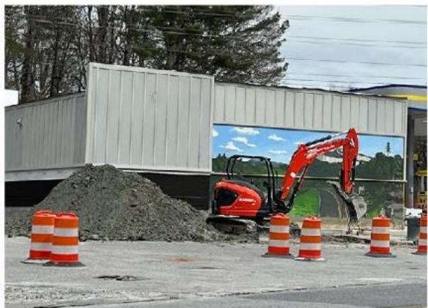
Flat Roof (inconsistent)
