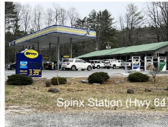
Spinix Station (Hwy 64) Accessory Structure Taller than Principal Building (inconsistent)
