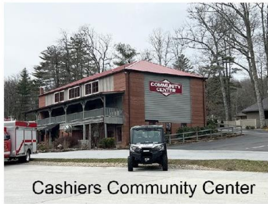
Cashiers Community Center 3-Story Building (inconsistent)
