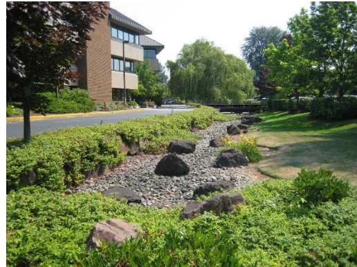
Figure 5. SEQ Figure \* ARABIC \s 1 1 Example of vegetated bioswale that catches and filters runoff
